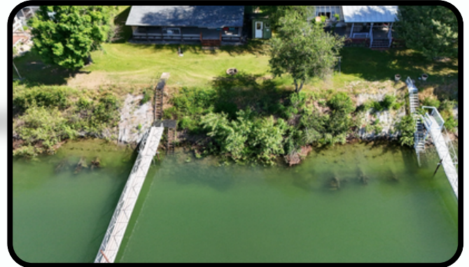
(Image 3. Sandy Shores Bank Stabilization Project Aerial View High Water Event within Project Reach May 2026)
